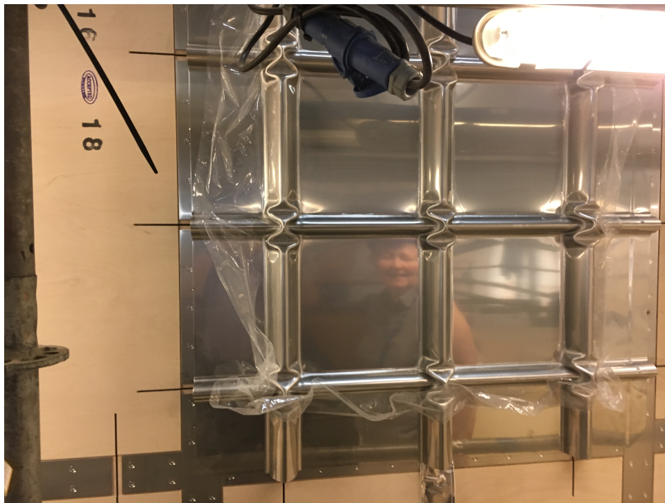
Membrane section installed on top of foam insulation inside the ProtoDUNE-SP cryostat.
