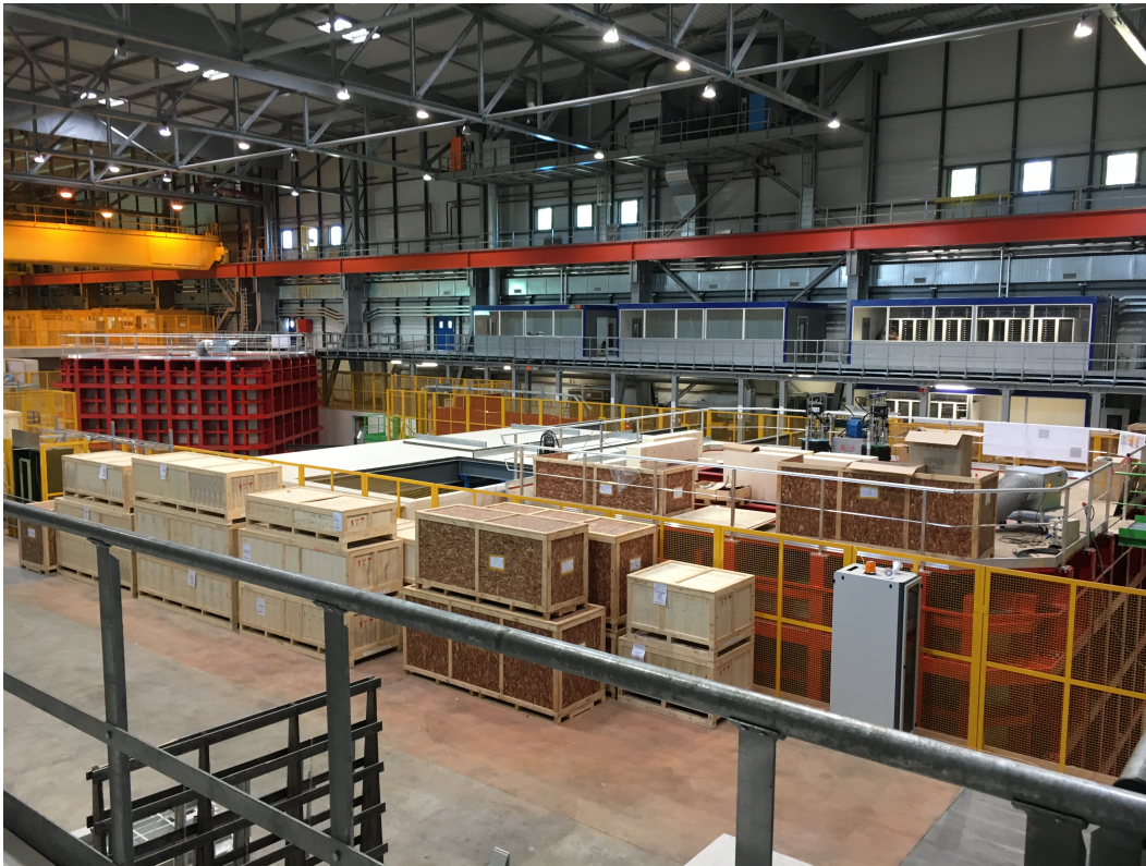
View of the CERN North Hall extension with the two ProtoDUNE cryostats now under construction. Some of the many boxes containing insulation and membrane cryostat parts are also visible.
